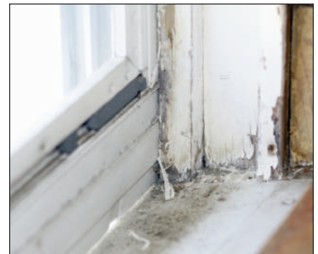
Opening and Closing Constantly Grinds Lead Dust
