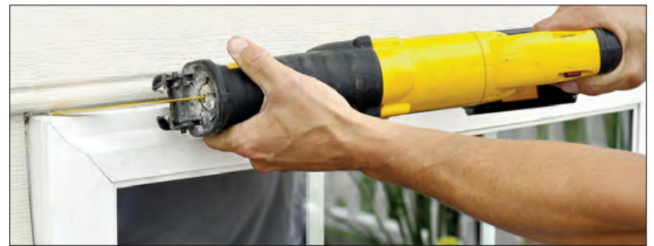
All pieces of the old wood framed window, complete with frame, sill and trim can be cut out to expose wall framing.
